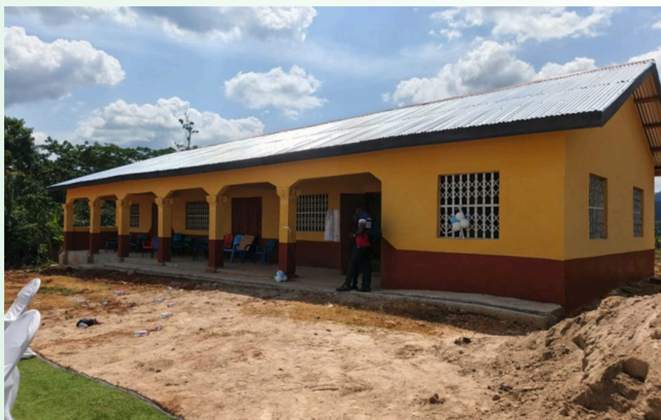
The 3-unit classroom block completed under "Oman Yie Die" at Owuratwum
